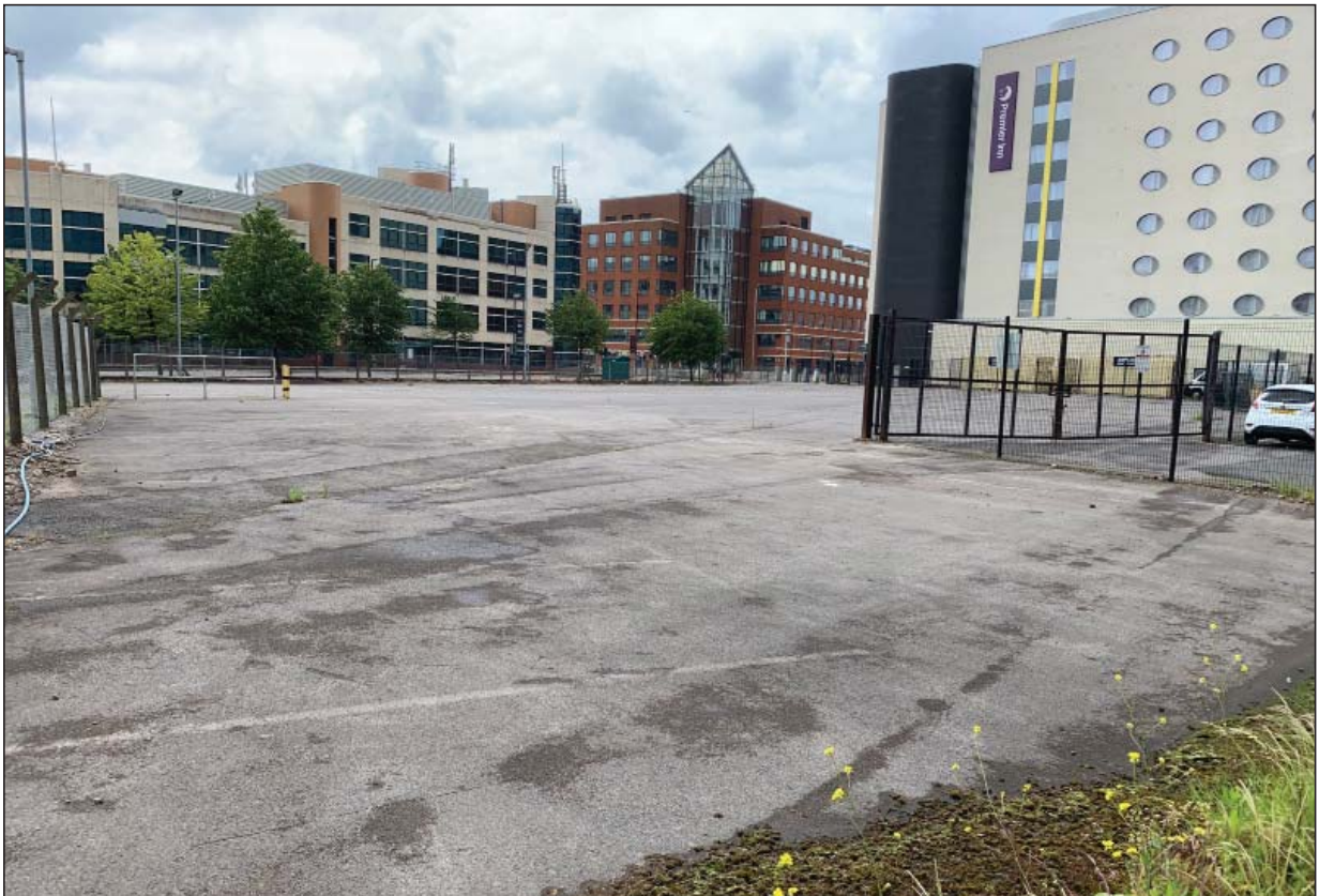
Plate 2 - Overview of Site, looking southwest
