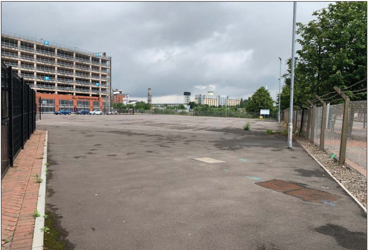
Plate 6 - Overview of south extent of Site, looking northeast
