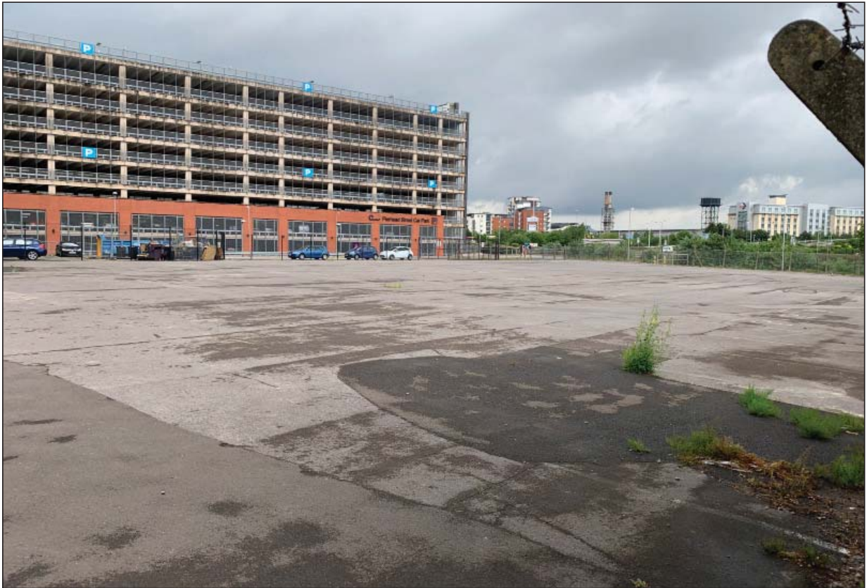
Plate 1 - Overview of Site, looking northeast
