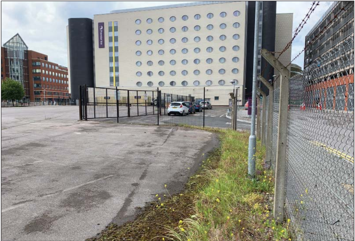
Plate 3 - Overview of north extent of Site, looking west-southwest
