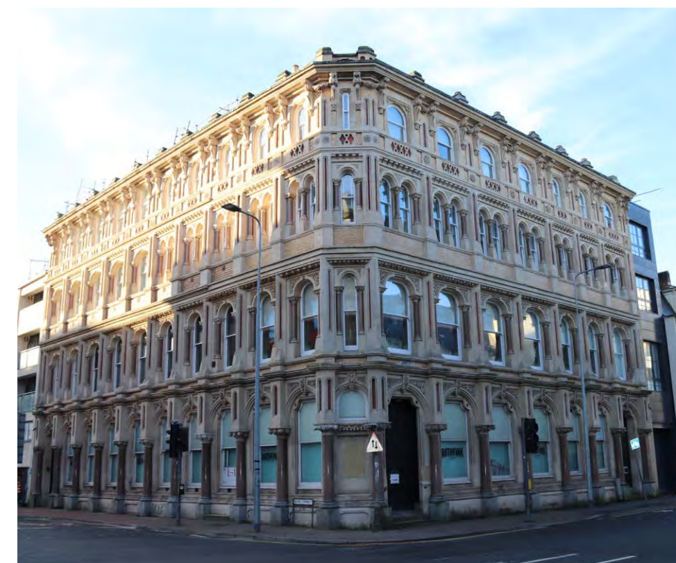
Former Cory Offices & then Midland Bank (source: own)
