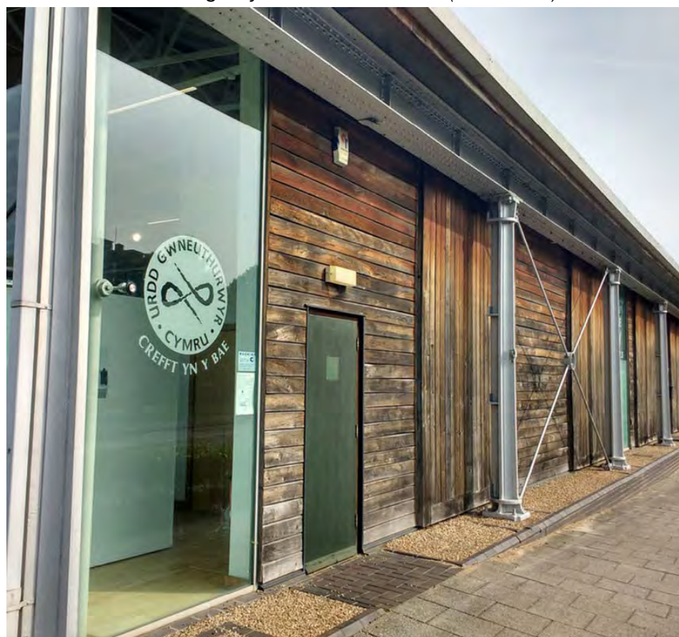
The Former Warehouse (The 'D' Shed), Craft In The Bay (source: 'makersguildinwales.org.uk')
