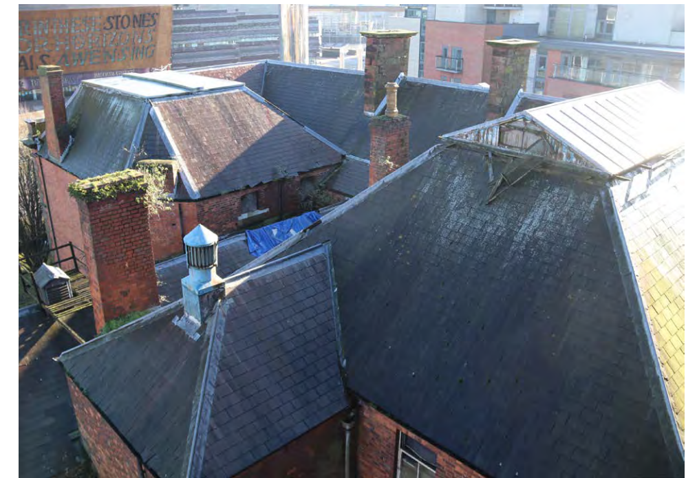
View of Roof from the Rear / North West
