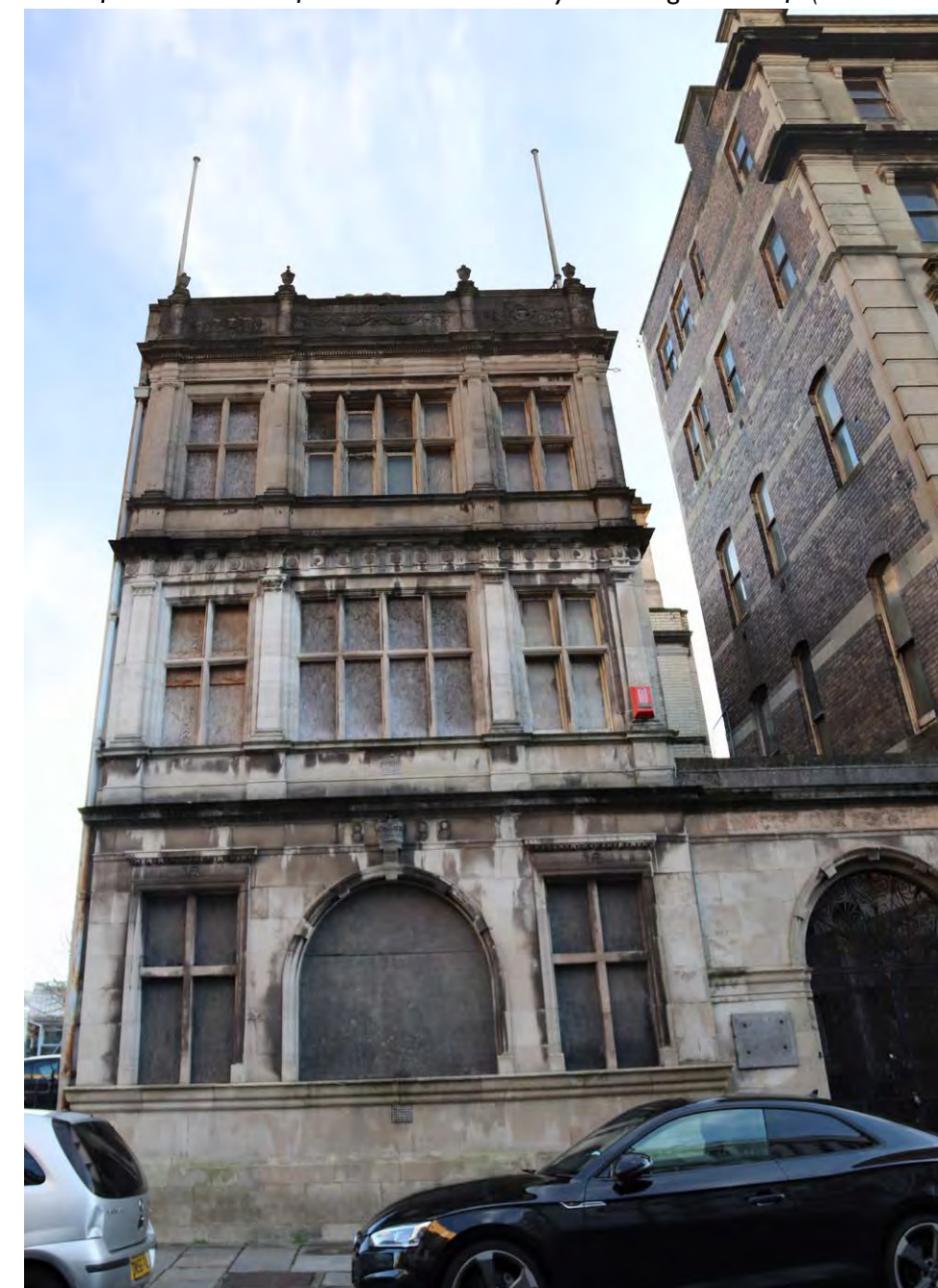
Custom House with Cory's Building to the right (source: own)
