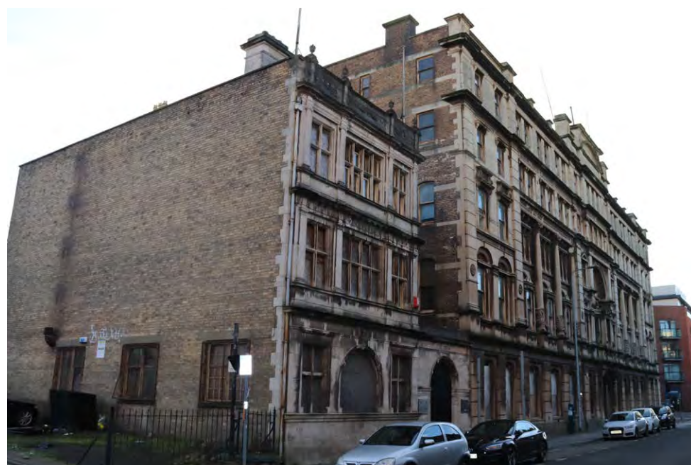
Custom House with Cory's Building to the right (source: own)
