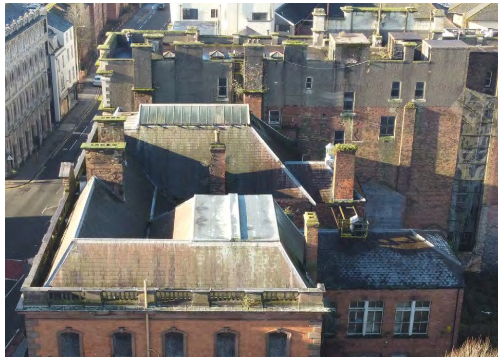
View of Roof from the Side / East
