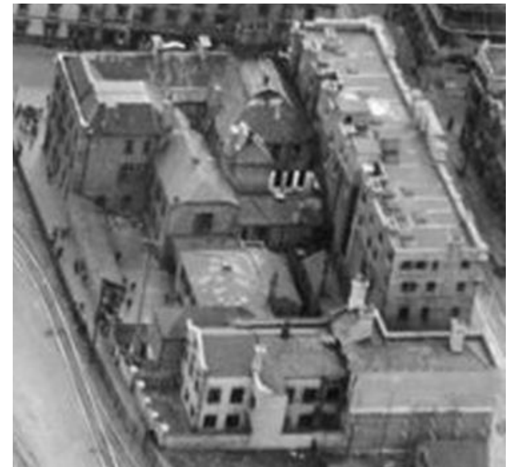
1929 Aerial photo of 'extended' top of Cory's Building (source: RCHAMW)
