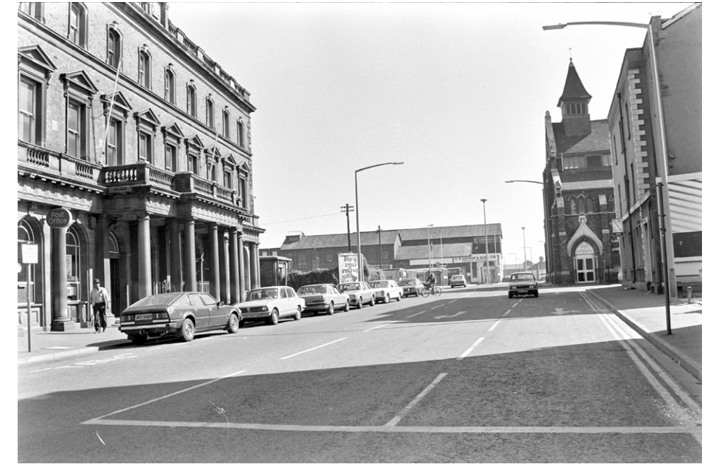
View of Merchant Place and Minton Treharne Building, Bute Place, with Mission to Seamen's Institute & Church at rear, 1982 (source: 'museum.wales')
