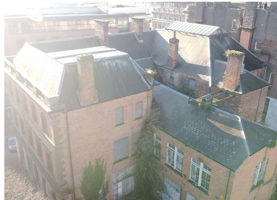
View of Roof from the Rear / North East
