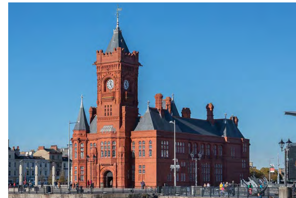
Pierhead Building as now (source: 'donaldinsallassociates.co.uk' website)
