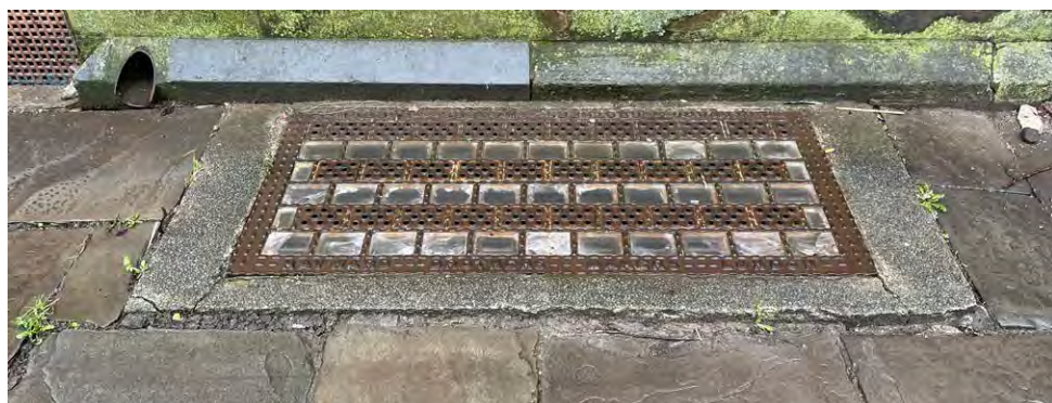
Above is the only pavement light still visible from above. All others have been covered over by the raised pavement at the front.
