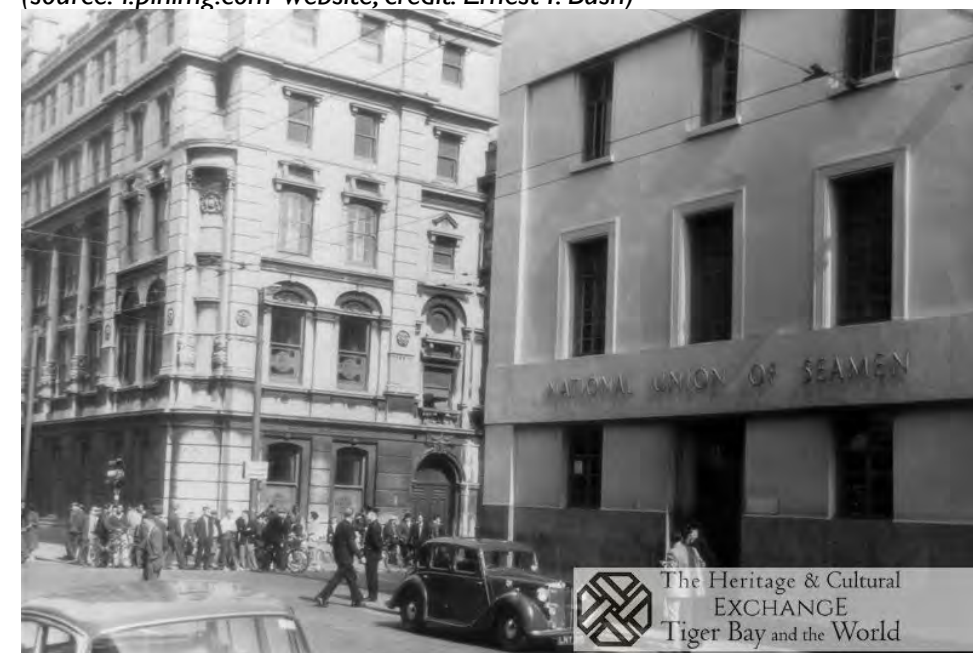
1950s Cory's Building with National Union of Seaman (source: 'hcearchive.org.uk')
