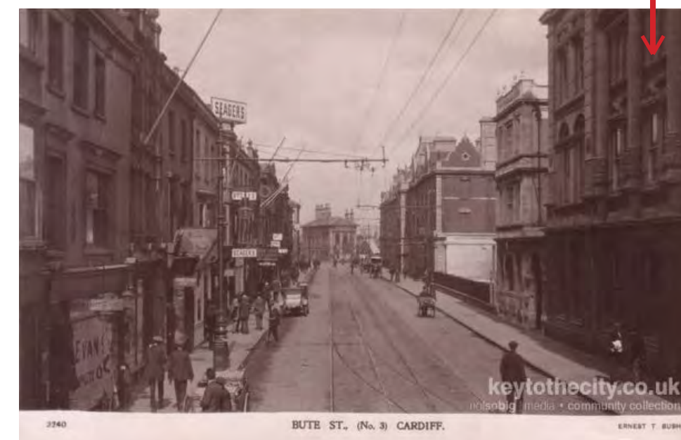
Bute Street in early 1900s with Cory's Building immediately to the right (identified by red arrow) (source: 'bing.com' website; credit: Ernest T. Bush)
