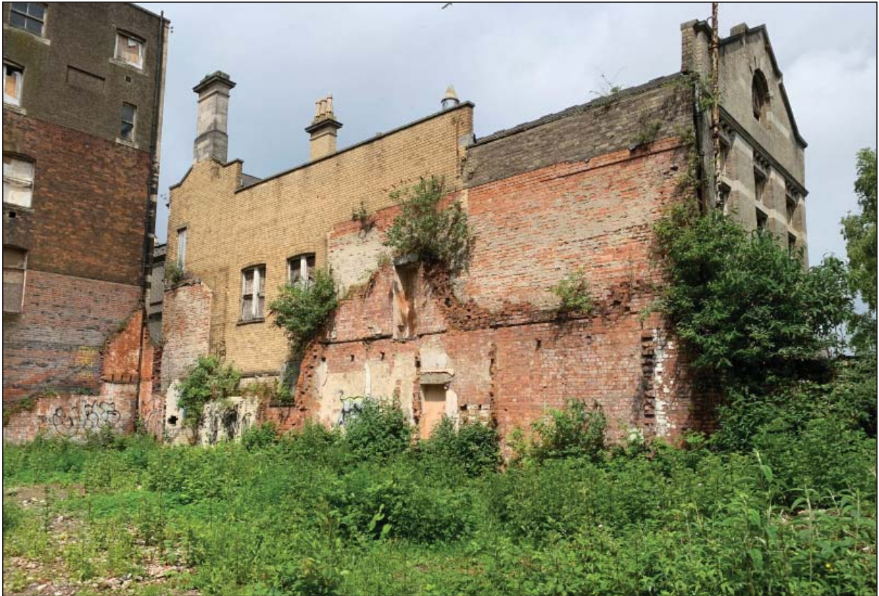
Plate 9 - North wall of courtyard showing evidence of previous abutting structures, looking northwest
