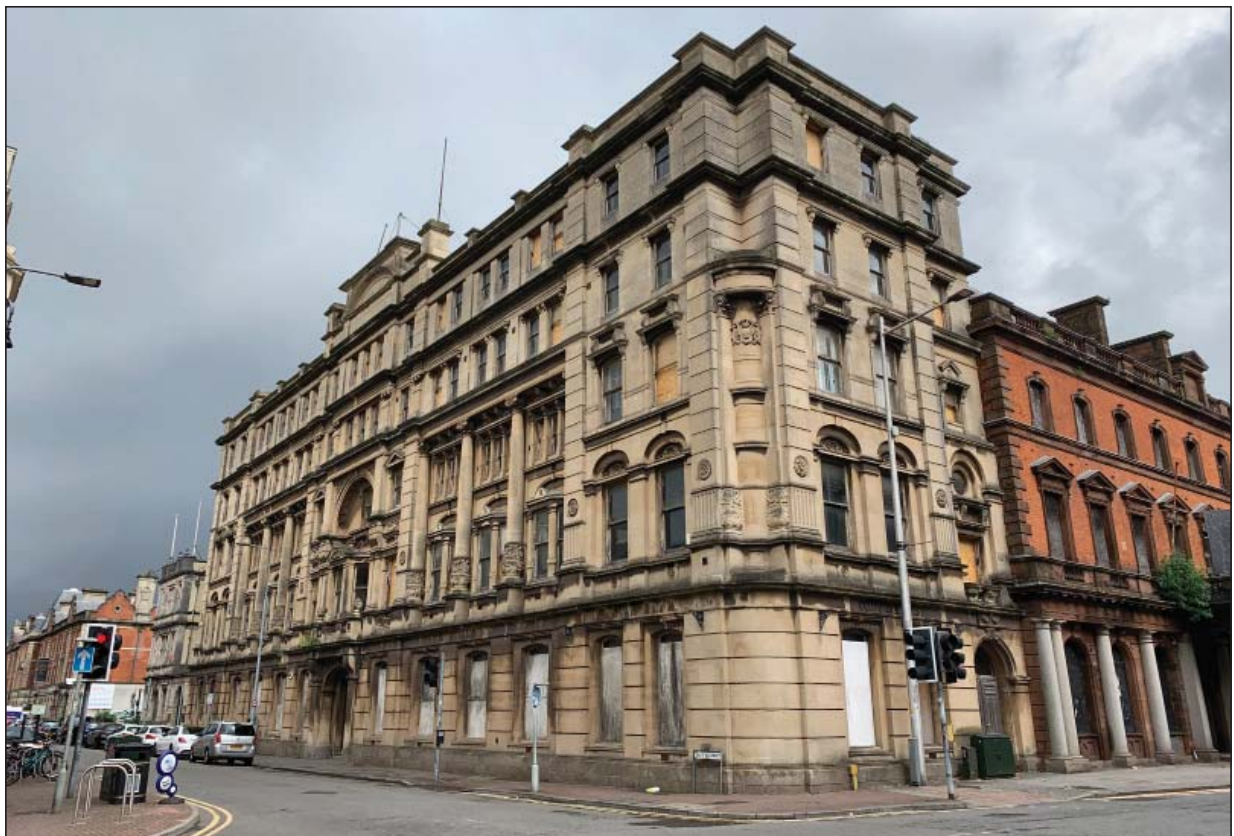
Plate 2 - Cory's Building, looking northeast
