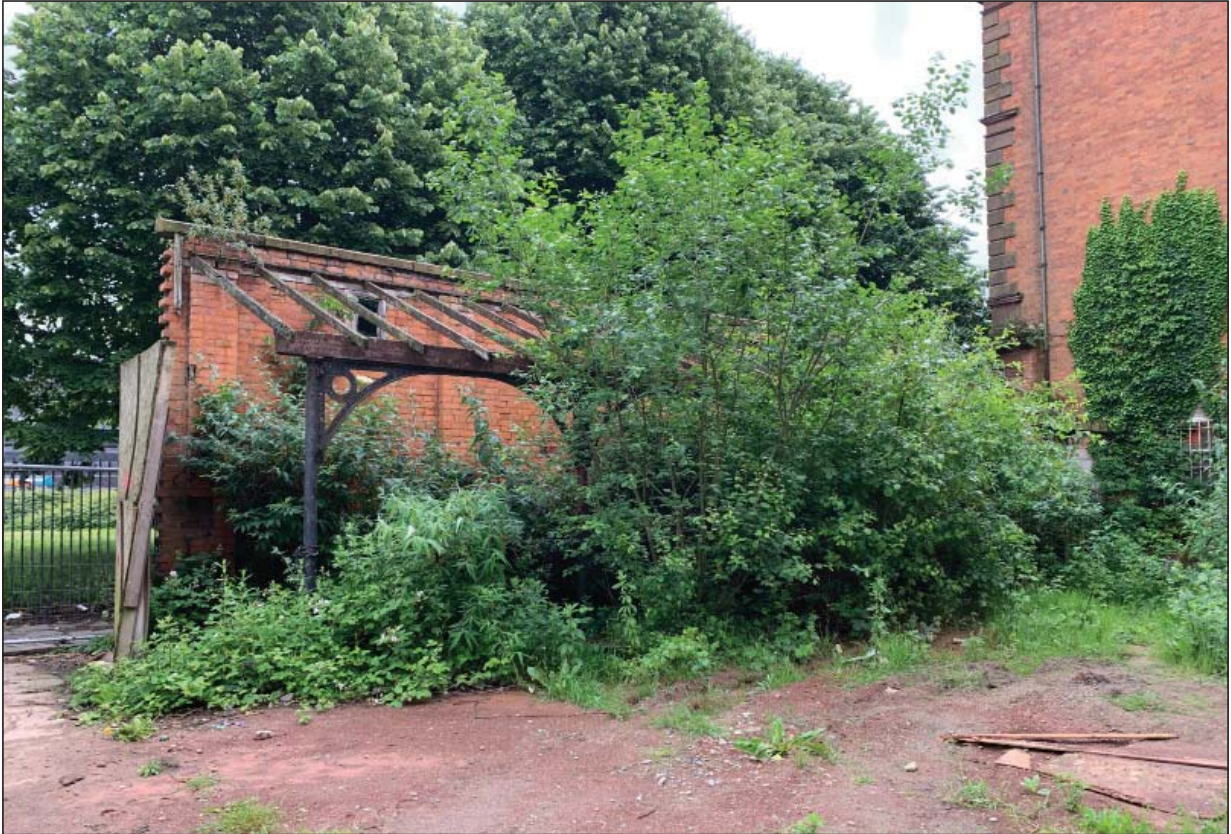
Plate 5 - Cast iron structure to south of courtyard entrance, looking southeast
