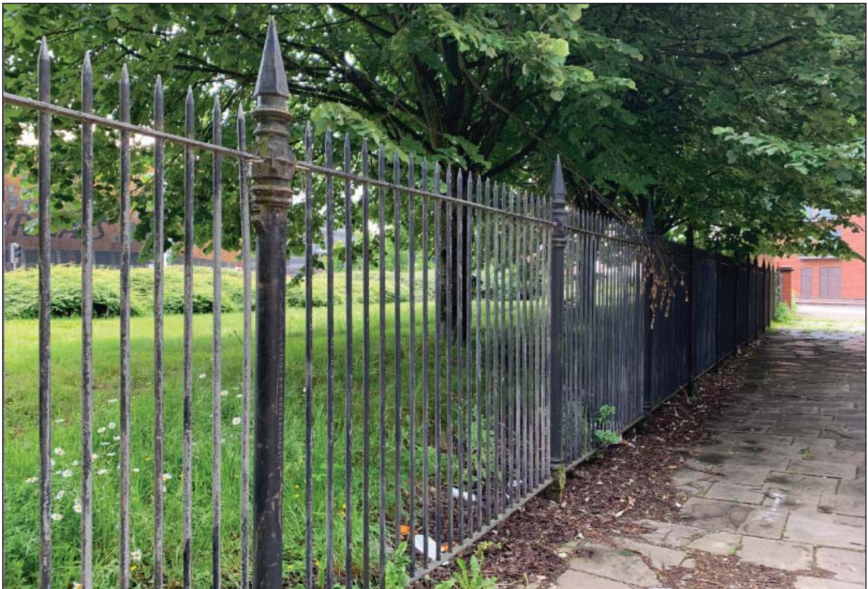
Plate 4 - Cast Iron Posts and Railings (LB 13985) beside courtyard entrance, looking southeast
