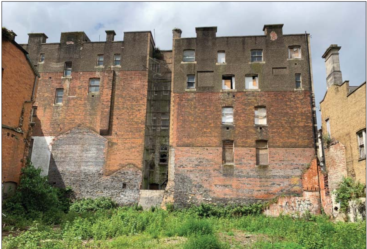
Plate 8 - Rear of Cory's Building showing evidence of previous abutting structures, looking west
