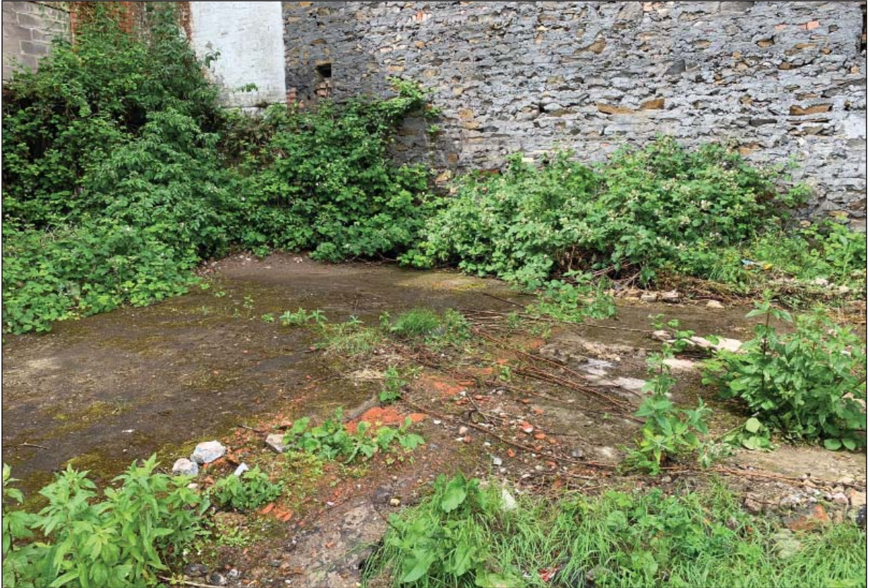
Plate 11 - Partial floor surface and wall foundations from previous structure, looking southwest
